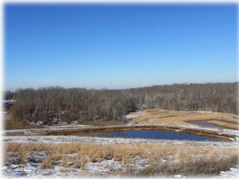
Figure 2: North-easterly view of the treatment system built at the Tab-Simco abandoned mine land site (Photo taken by author, February 2013).
